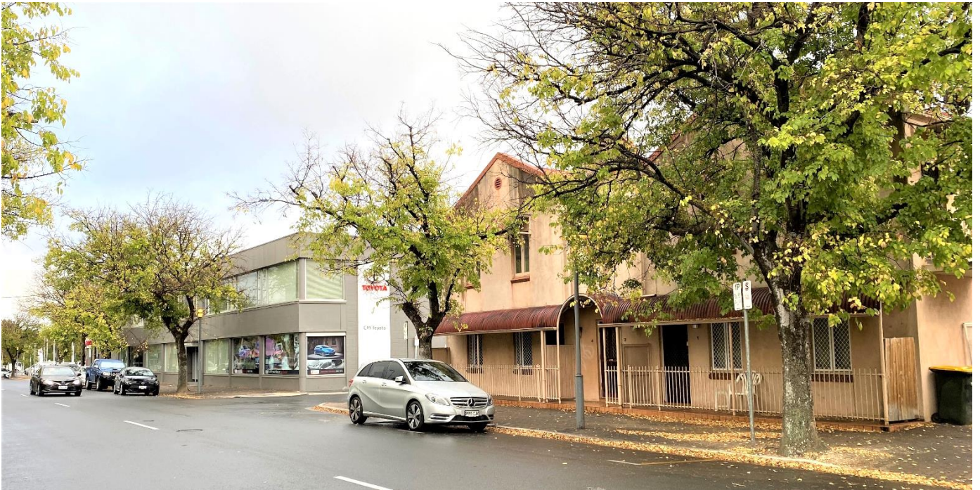
Photo 3 – Northern side of Tynte Street looking west to west Terrace with a mix of residential and commercial premises
