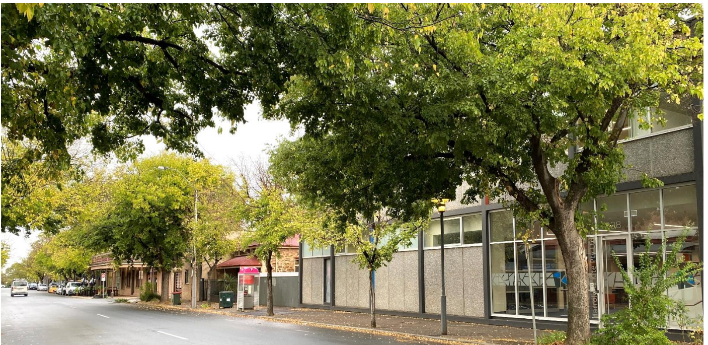
Photo 4 – Northern side of Tynte Street looking west with the Prince Albert Hotel visible in the background on the left and a commercial premises in the foreground.
